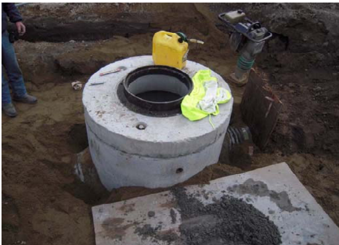
Figure 3 – Silt and Grease Trap (water quality treatment unit – Scotts Valley Library)
